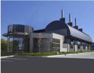
New Boiler House
