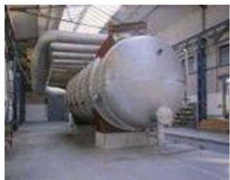
Evaporator set in place
