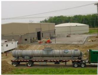
Evaporator heat exchanger being moved into the building
